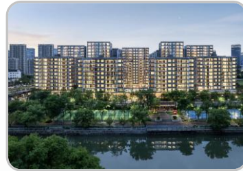
Quality delivery of Zhejiang's first general contracting construction project - Hangzhou Xiaofeng Langyue
